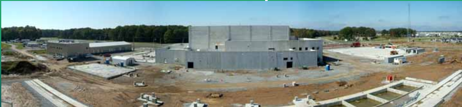
Paducah Conversion Facility, October 2006
