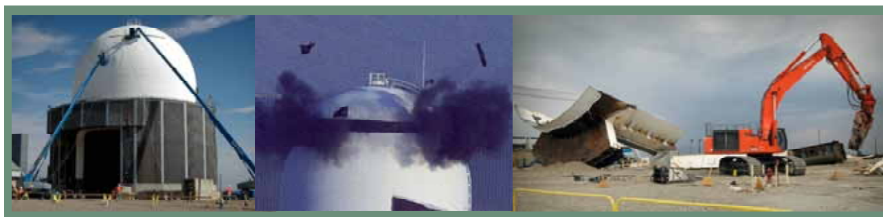
Fig. 4. Test Area North 650 and 630, where the Loss of Fluid Test Facility was demolished.
