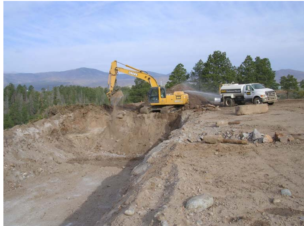
Excavation of contaminated absorption bed fill material
