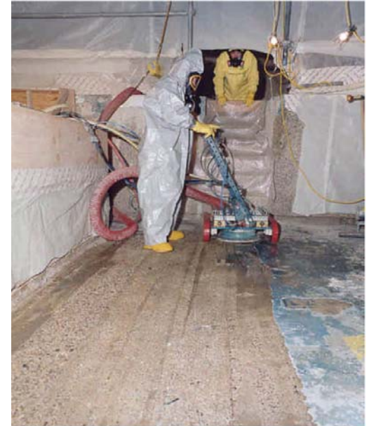
Hydroblasting in B-707
