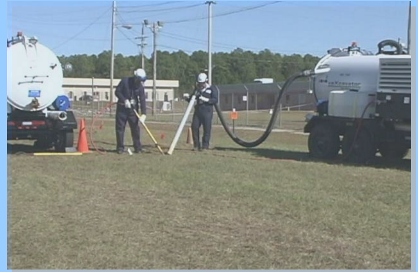
Vacuum Excavator improves electrical safety
