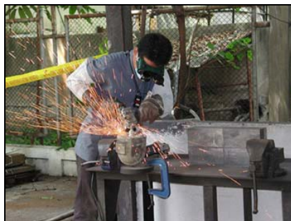
Fig. 1. Weld cutting using electrical blade
