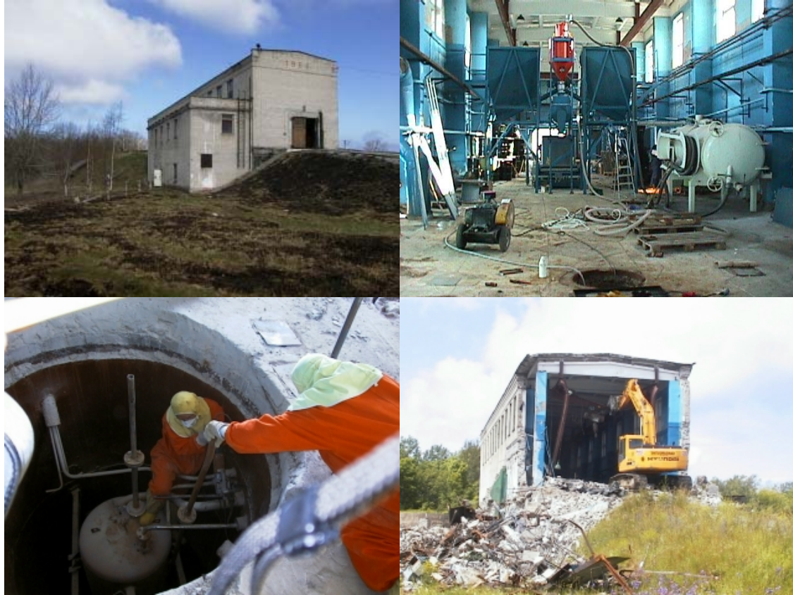
Fig. 3. The Liquid Waste Storage (LWS)
