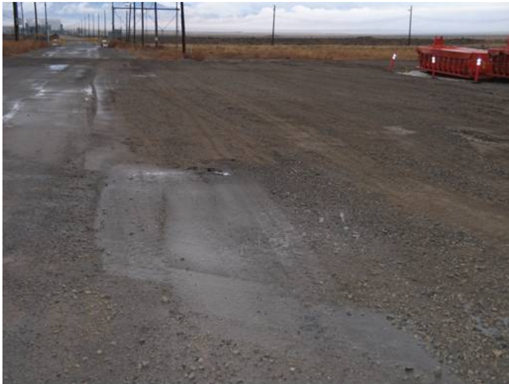
Fig. 5. Real-time remediation process showing post-excavation survey and the backfilled area.
