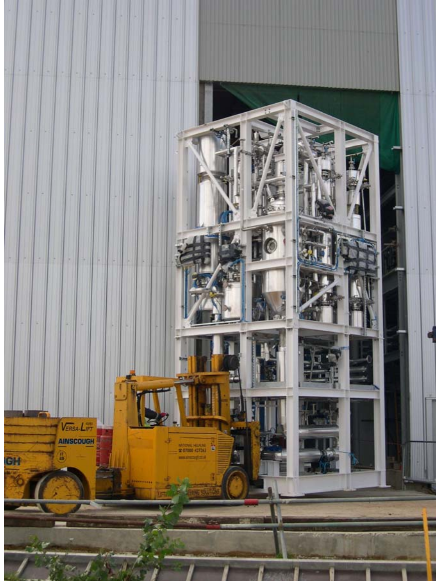
Fig. 2. One of the Evaporator Modules Being Installed into the WTP
