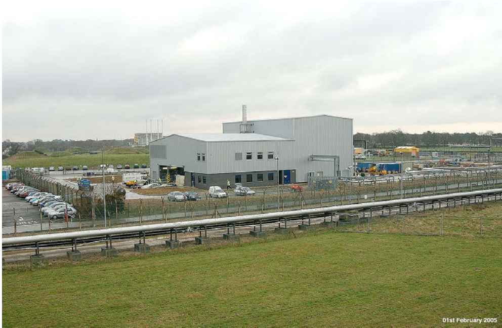
Fig. 1. WTP during construction
