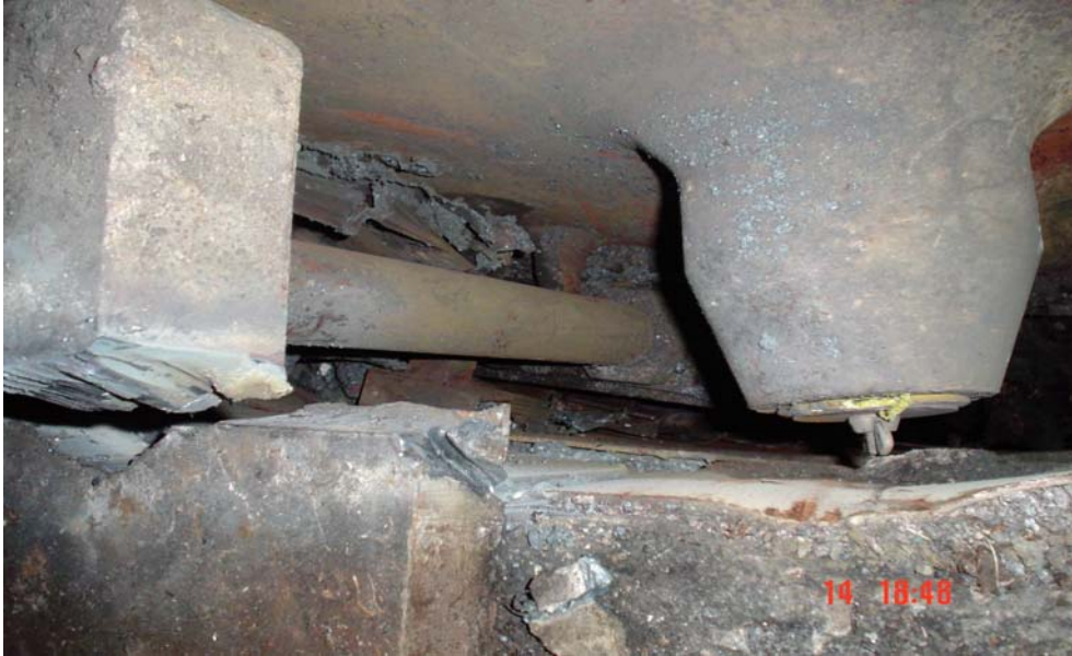
Fig. 1. Clearance between reactor vessel and cavity wall
