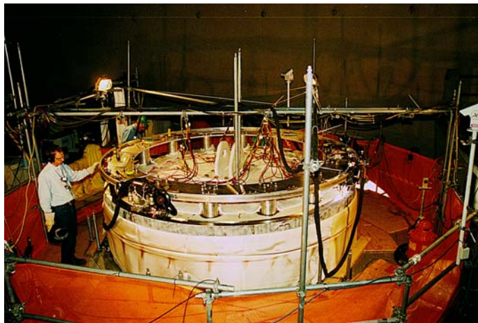
Fig. 3. Welding of the reactor vessel container lid
