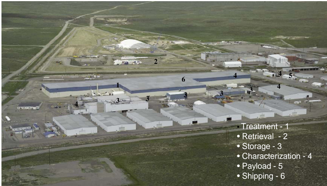
Fig. 1. Advanced Mixed Waste Treatment Facility
