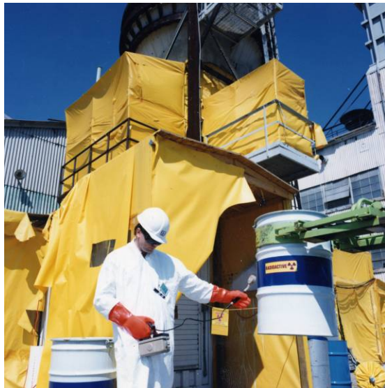
Fig. 3. Drummed waste being surveyed for transportation
