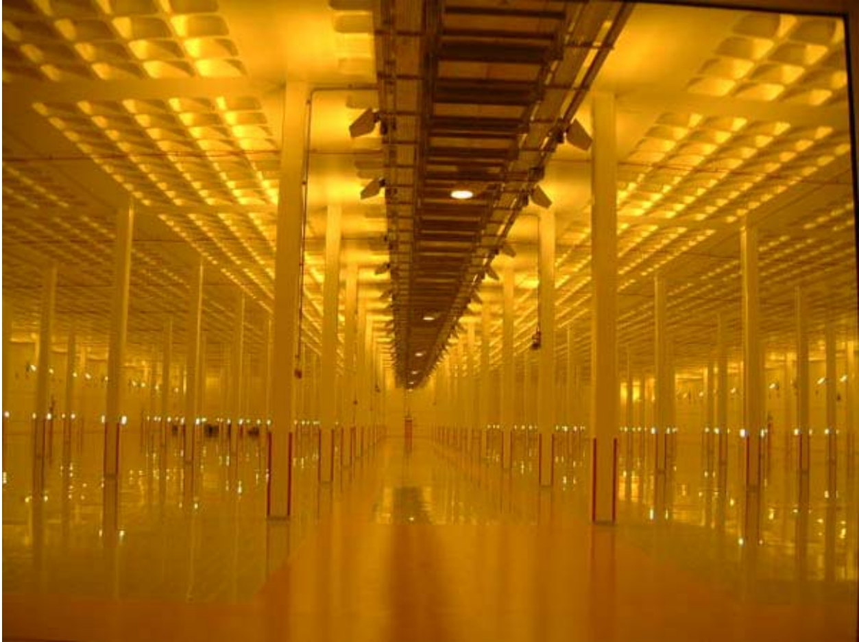
Fig. 3. Inside the recently constructed Engineered Drum Store 3
