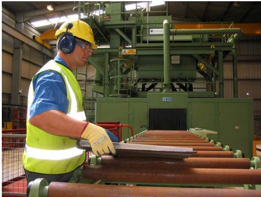
Fig. 2. Wheelabrator at the new Sellafield Metals Recycling Facility
