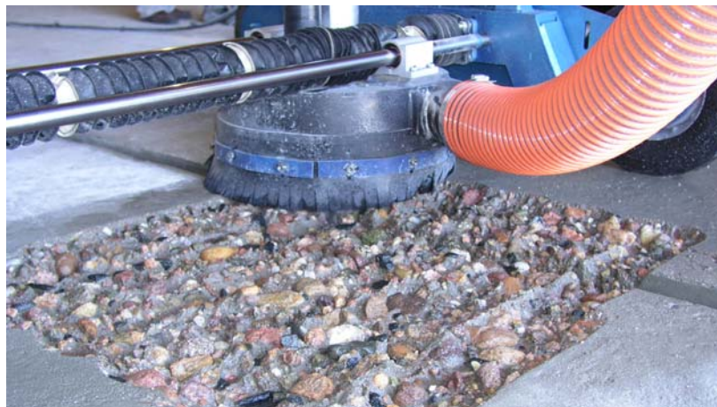
Fig. 1. Remote hydrolasing to remove concrete surfaces
