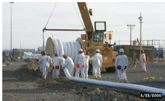
Fig. 3. The hose in hose sludge transfer system, cross section and installation
