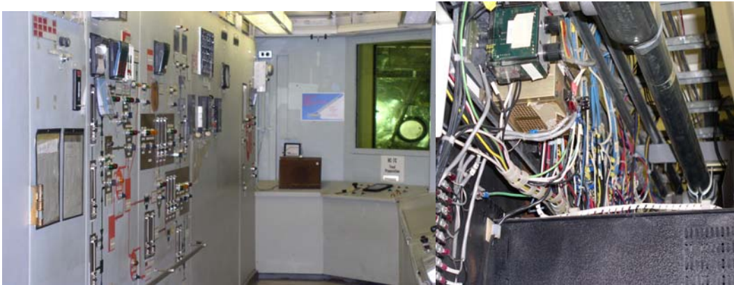
Fig. 4. Front and back view of control panels
