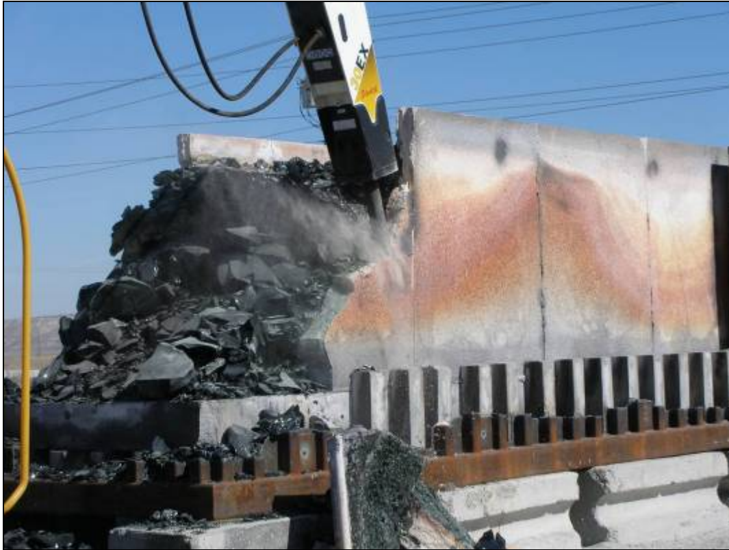
Fig. 7. Post-melt ICV™ container examination and dismantling
