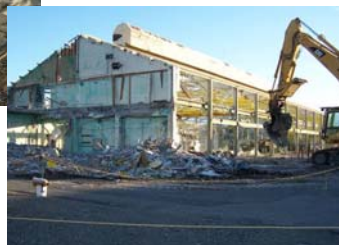
River Corridor building demolition
