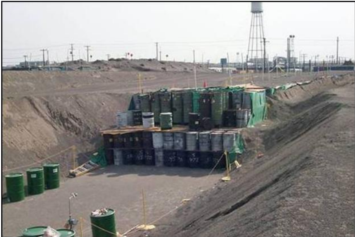
Fig. 1. TRU storage module, burial ground 218-W-4C.
