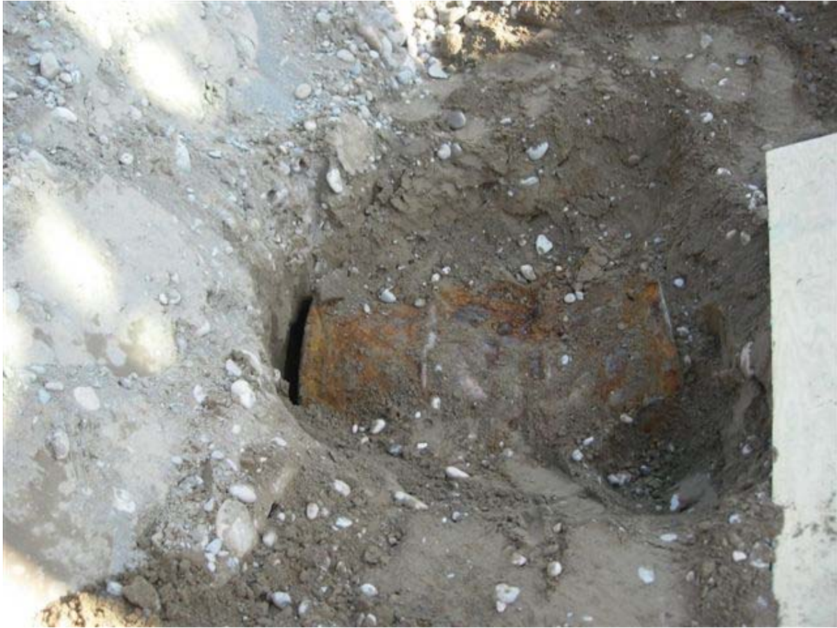
Fig. 4. Direct buried suspect TRU drum in burial ground 218-E-12B.
