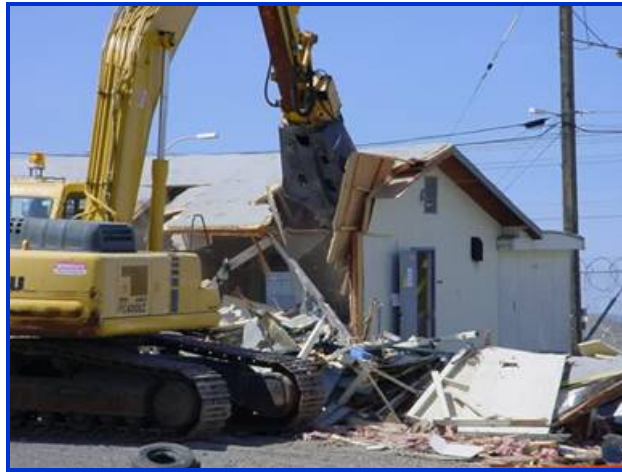
Fig. 3. A typical ancillary facility is undergoing demolition.
