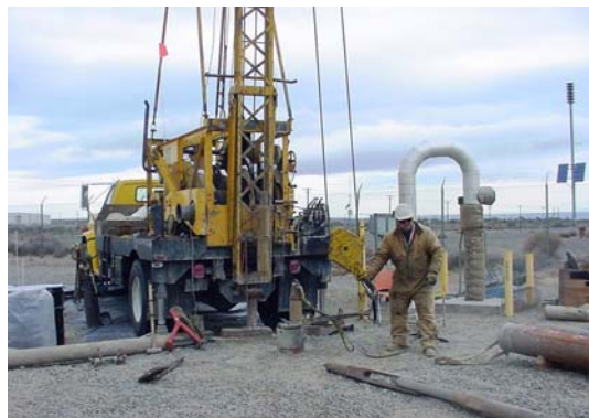
Fig. 4. Wells are drilled on the central Hanford Plateau to extract contaminated water.
