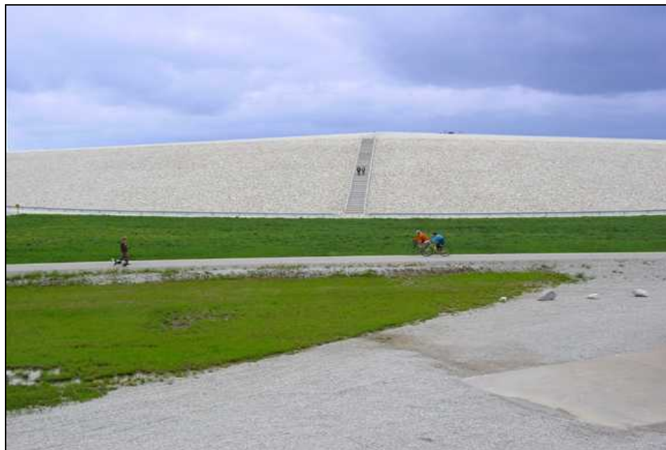
Fig. 3. The Hamburg Trail and ramp to the top of the disposal cell
