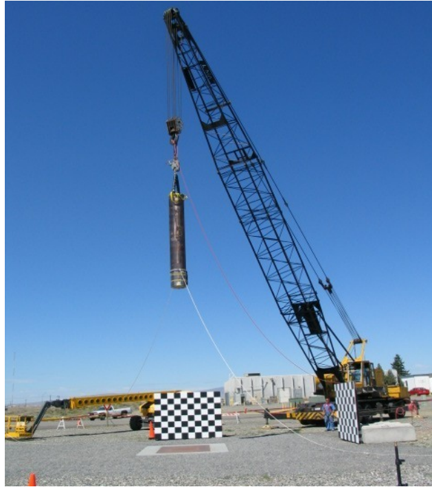
Fig. 4. Thin-walled canister staged for the drop test
