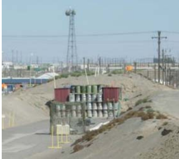
Fig. 2. Burial Trench showing four tiers of waste containers
