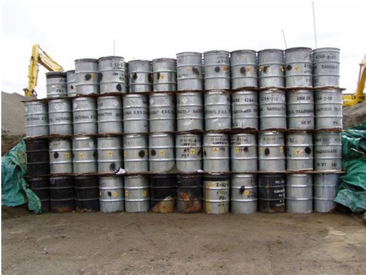
Fig 1. Typical TRU module in the 218-W-4C burial ground
