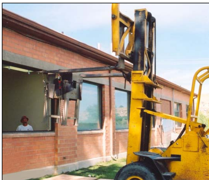
Fig. 3. Removal of a germanium detector unit from the Analytical Chemistry Laboratory
