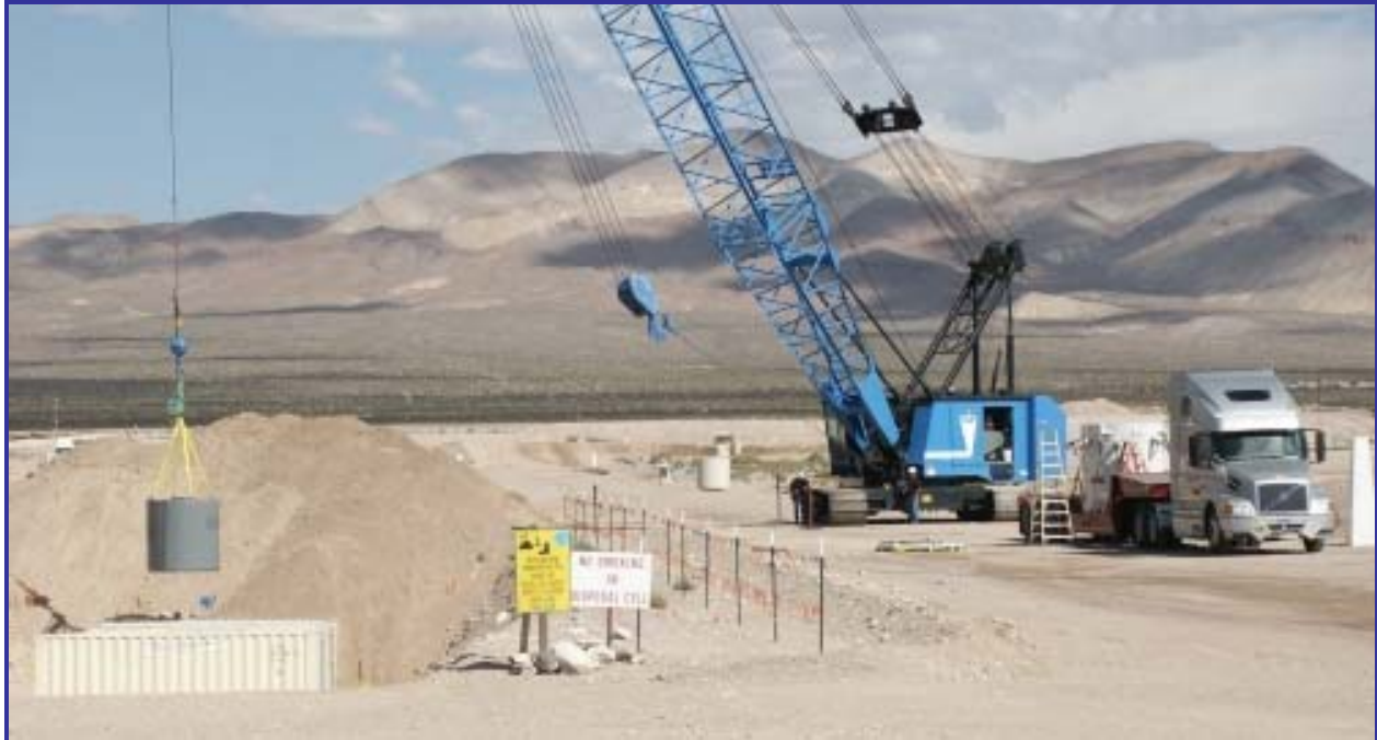
Fig. 3. A Foster-Wheeler high-activity LLW monolith being disposed at the Area 5 RWMS
