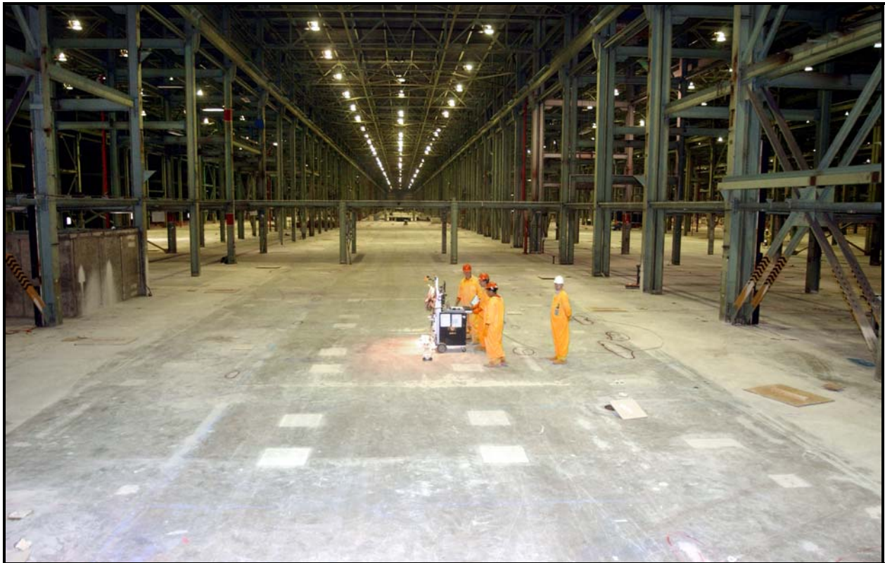
Fig. 3. SCM Survey of Floors in K-33
