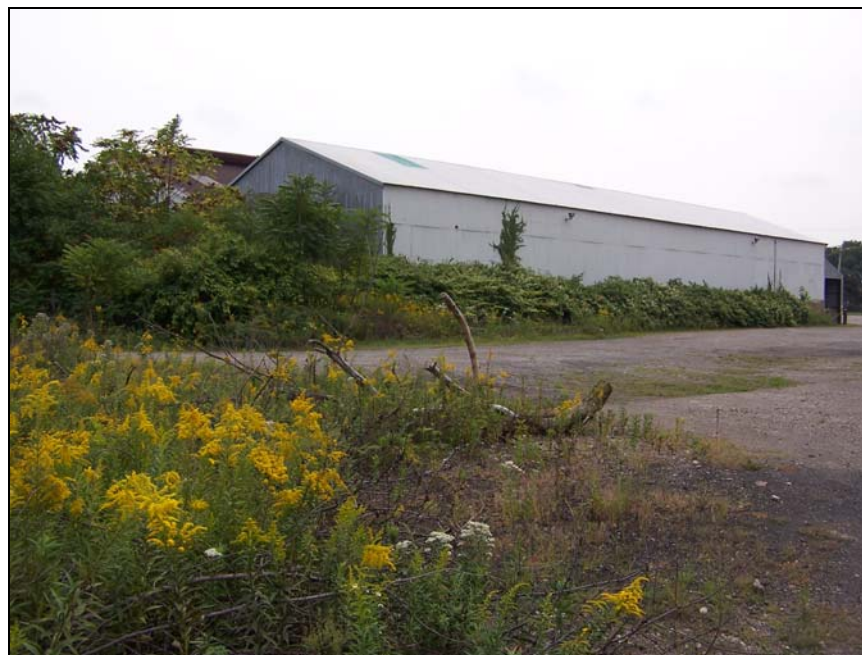
Fig. 3. Aliquippa, Pennsylvania, site, September 2005
