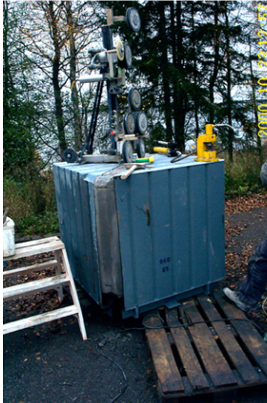
Fig. 3. Method of cutting through the sheet-metal container diagonally
