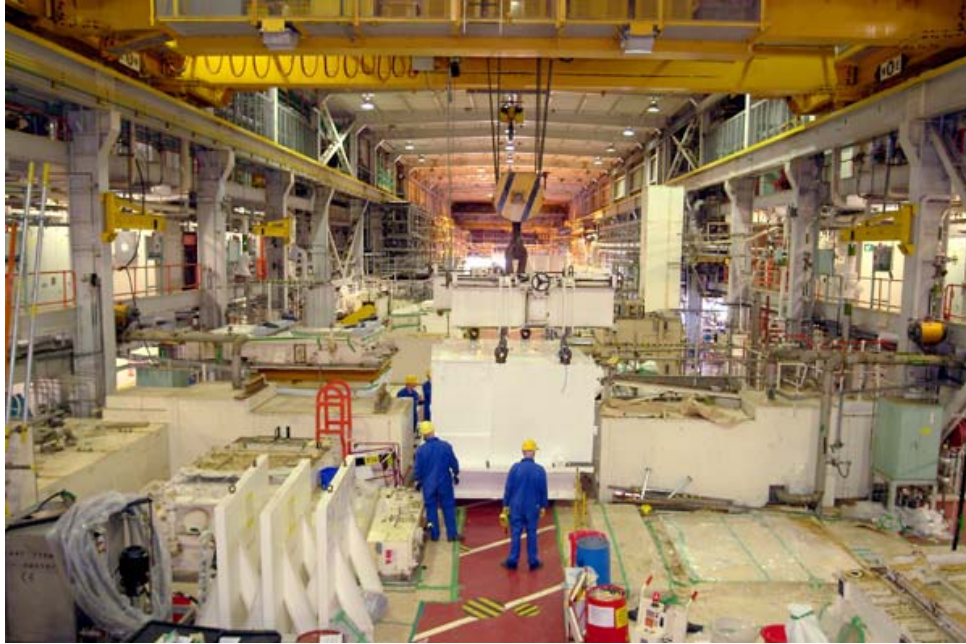
Fig. 1. SRF 45-ton module being removed from the silo operating floor
