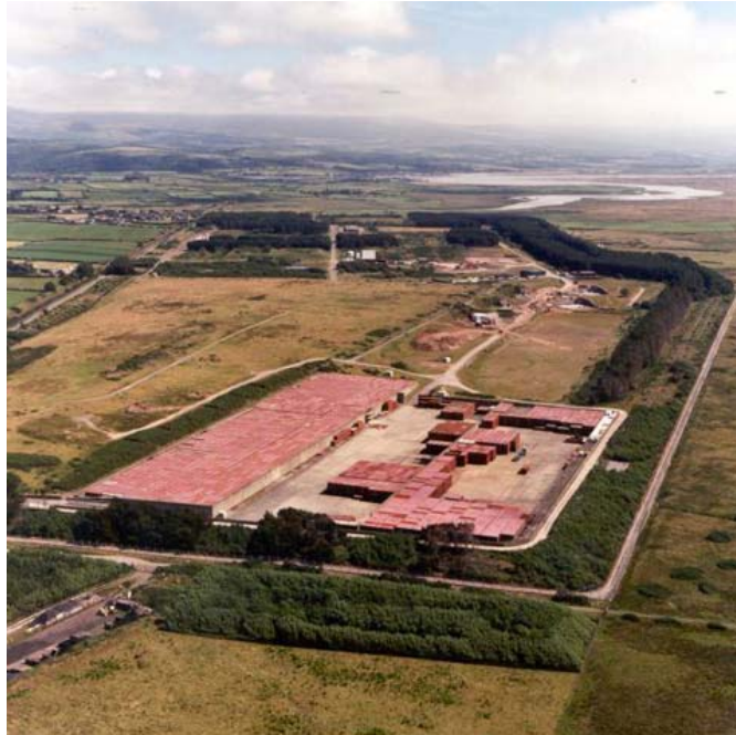
Fig. 2. National asset – the UK's only Low-level Waste Repository
