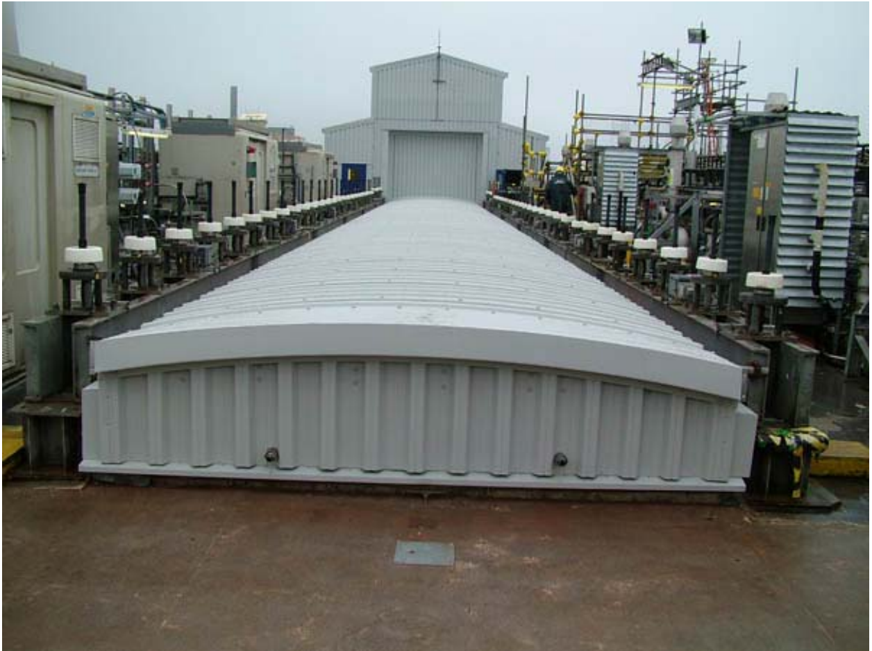
Fig. 4. View following total demolition and capping of the Transfer Tunnel
