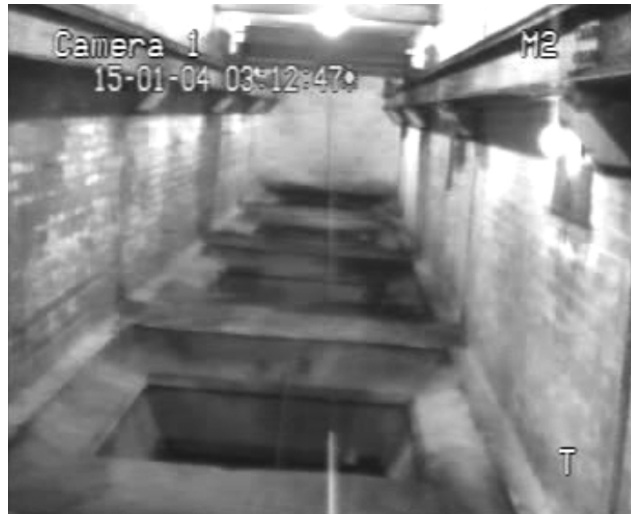
Fig. 3. View inside the transfer tunnel upon completion of waste clearance work.
