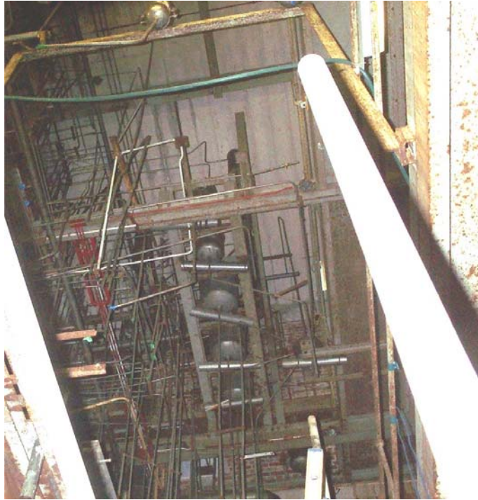
Fig. 4. Progress in the north cell mid-2005
