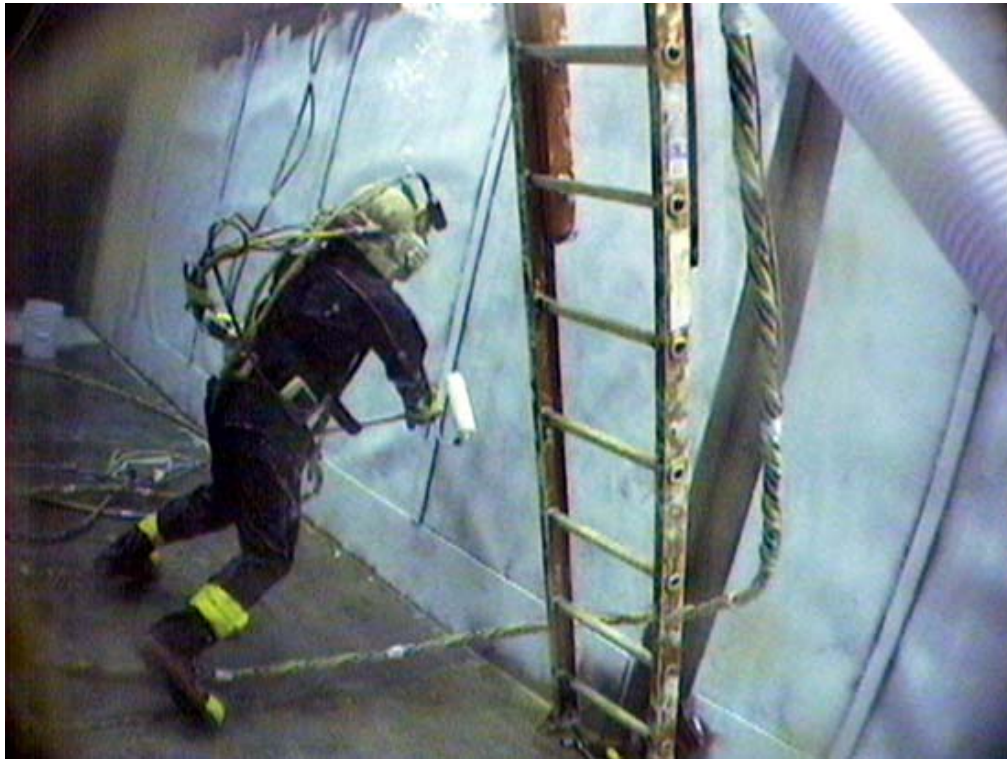
Fig. 2. Special two hose roller system used for wall coating
