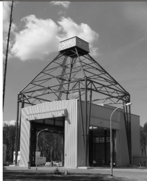
Drop tower with closed test building
