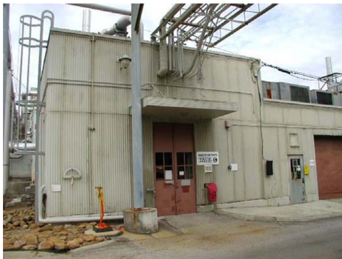
Fig. 2. Exterior of a typical building along "Isotope Circle"
