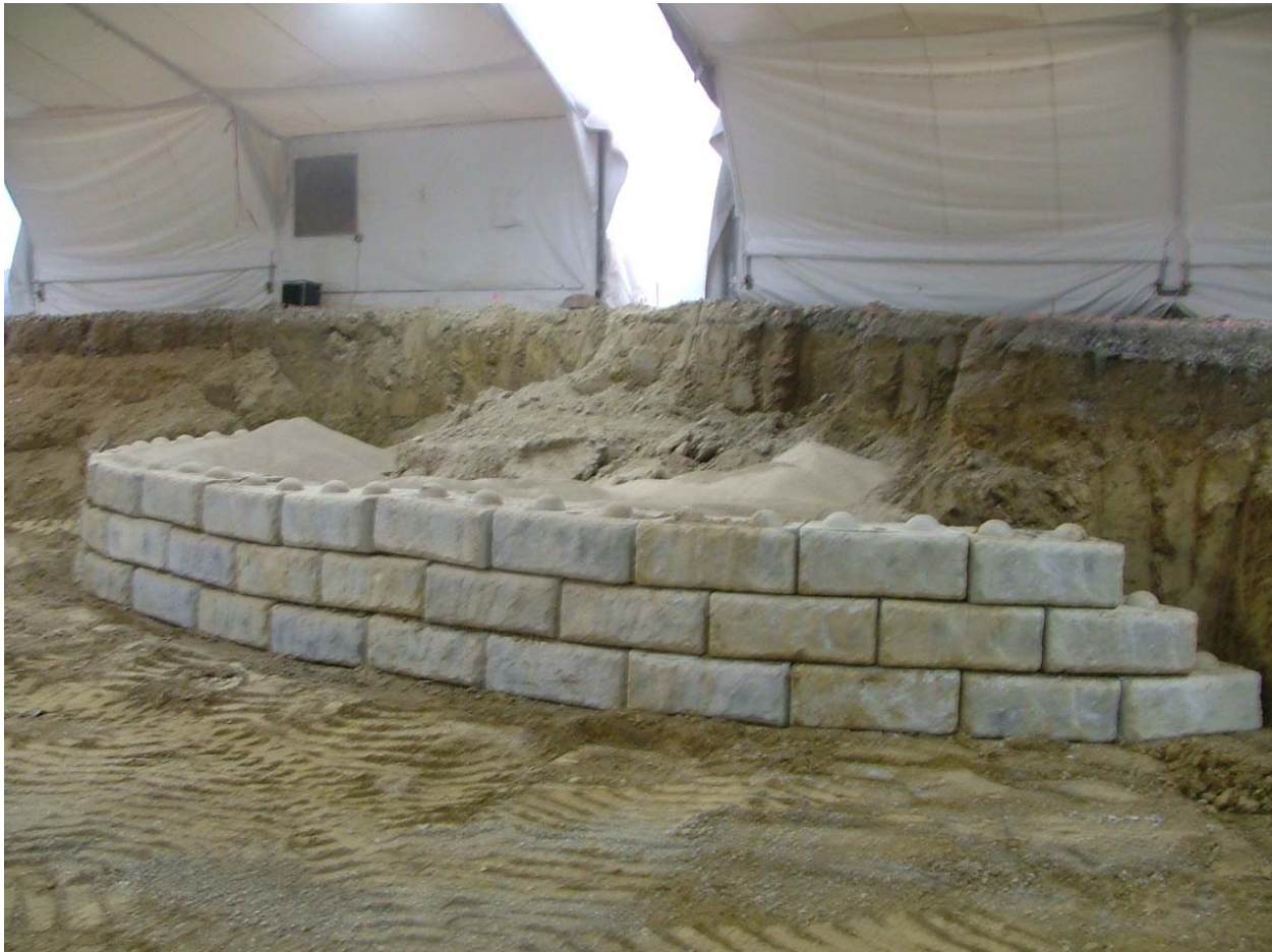
Fig. 2. Stabilization of Trench 13 area
