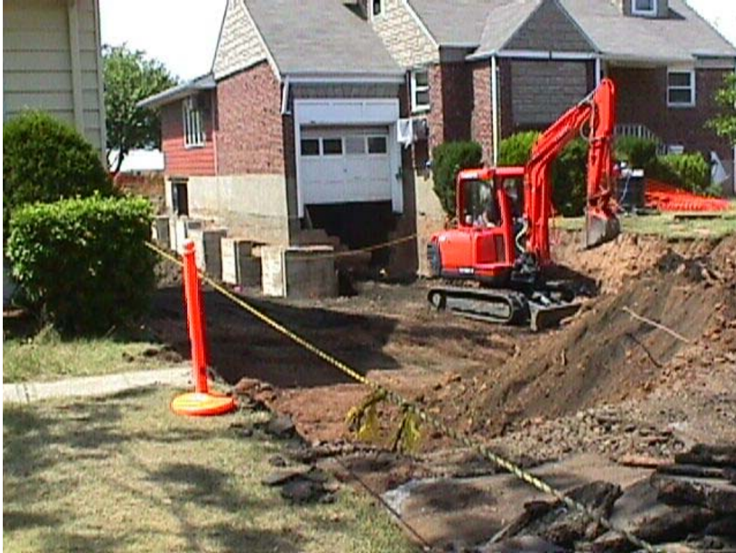
Fig. 4. A remedial construction effort is underway at this residential property in 1998.
