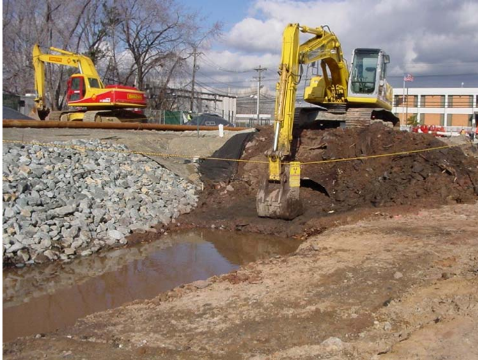
Fig. 5. This photo shows remedial construction at a commercial property in 2003. The process of removing contaminated soil displaced most of the employee parking at the site, requiring provision of temporary parking by the project.
