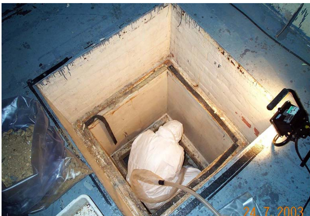
Fig. 3. Removal of contamination from below ground filter pit
