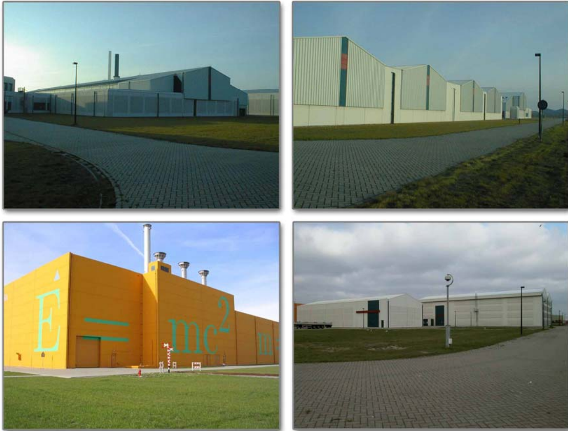
Fig. 2. The different buildings at the COVRA site, clockwise: building for waste treatment (upper left), for storage of low and intermediate level waste, NORM waste, and high level waste (lower left).
