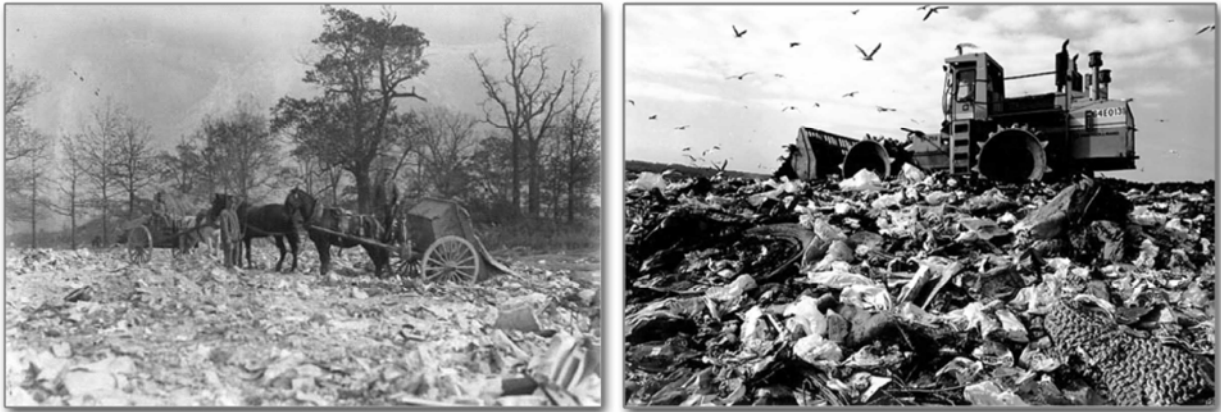
Fig. 1. Disposal of waste in New York around 1900 (left) and 2000 (right).[4]
