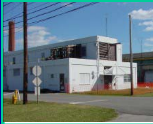
Building 1301 at East Tennessee Technology Park (ETTP)
