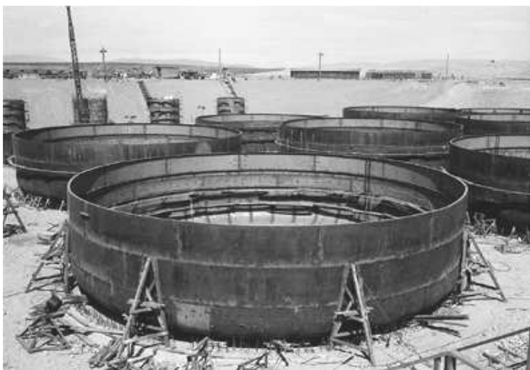
Fig. 1 One of Hanford's single-shell tanks during construction
