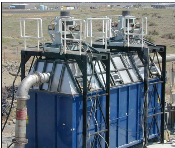
Fig. 7. Photograph of a 28-m 3 (37-yd 3 ) melt container and off-gas hood assembly during a full-scale Bulk Vitrification test.
