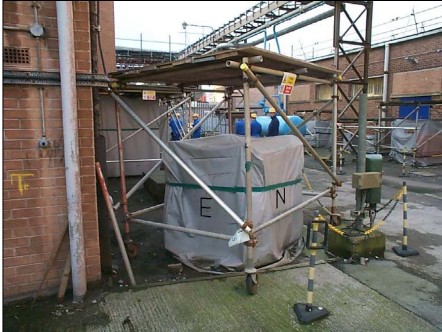
Fig. 2 A crated waste item in the compound
