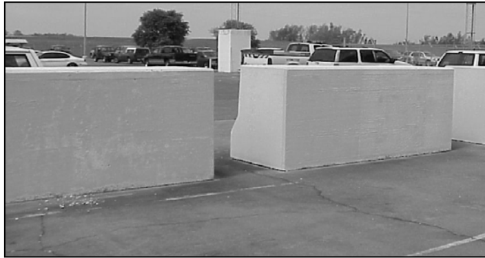
Fig. 2 Man-made concrete inertia barrier
