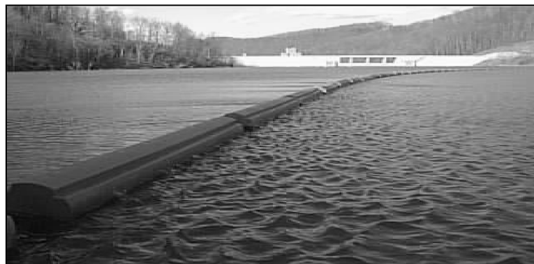
Fig. 3 Representative Watercraft deterrent barrier
