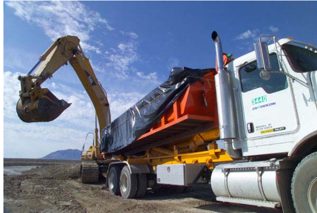
Fig. 1 Contaminated soil is excavated from a site at the INEEL
