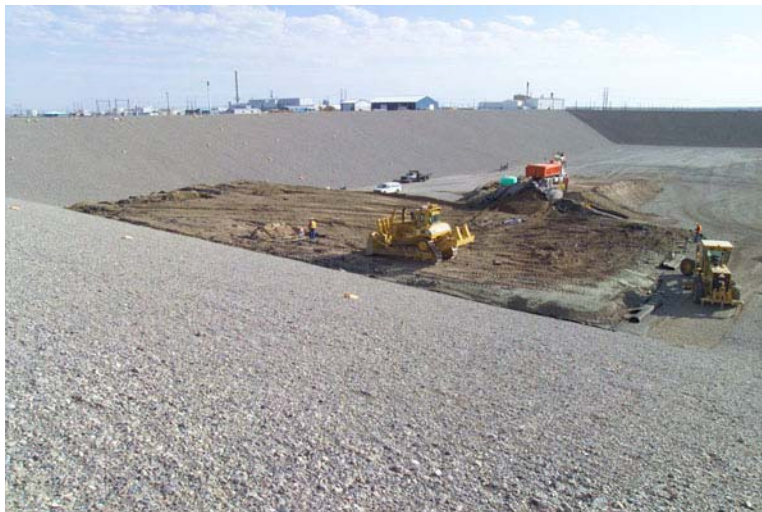
Fig. 3 Contaminated soil is placed in the landfill cell and compacted
