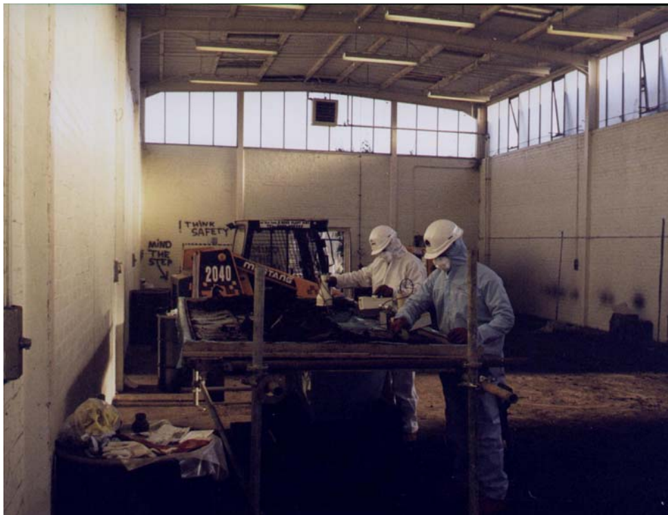
Fig. 4 Monitoring and segregation of waste exported offsite for disposal, particularly to Drigg as low level waste.
