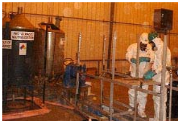
Fig. 1 Workers decontaminating a silver recovery unit.
