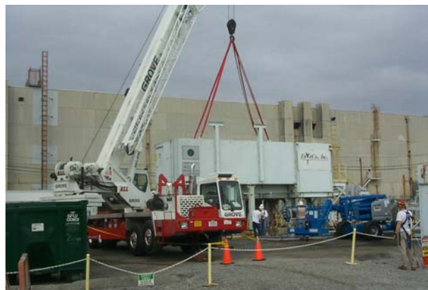
Fig. 3 TVS dismantlement activities
