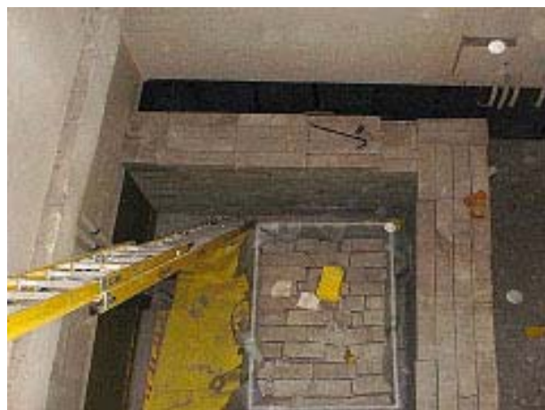
Fig. 2 Segregation of barite shield blocks
