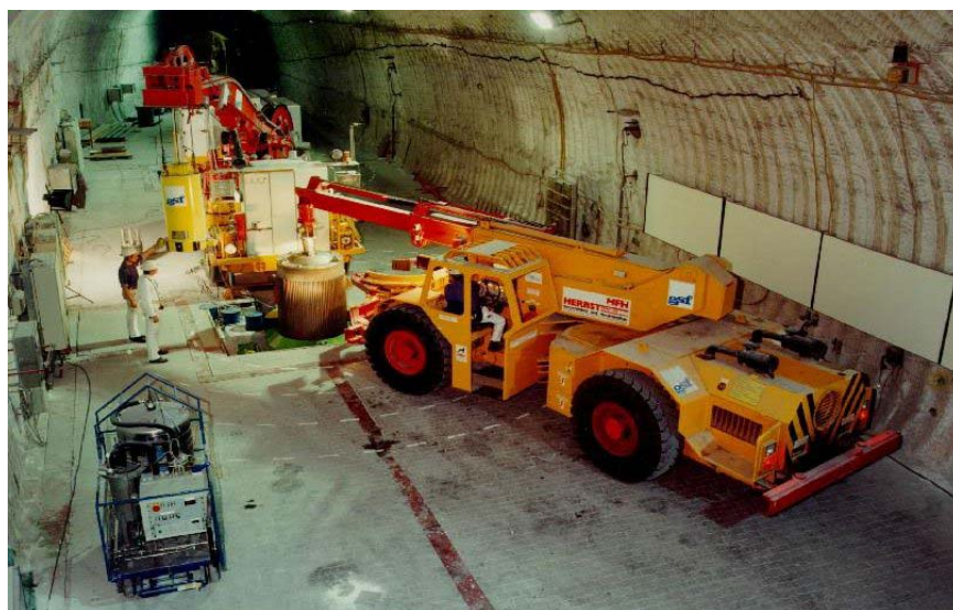
Fig. 5 HAW-Project test site during construction
