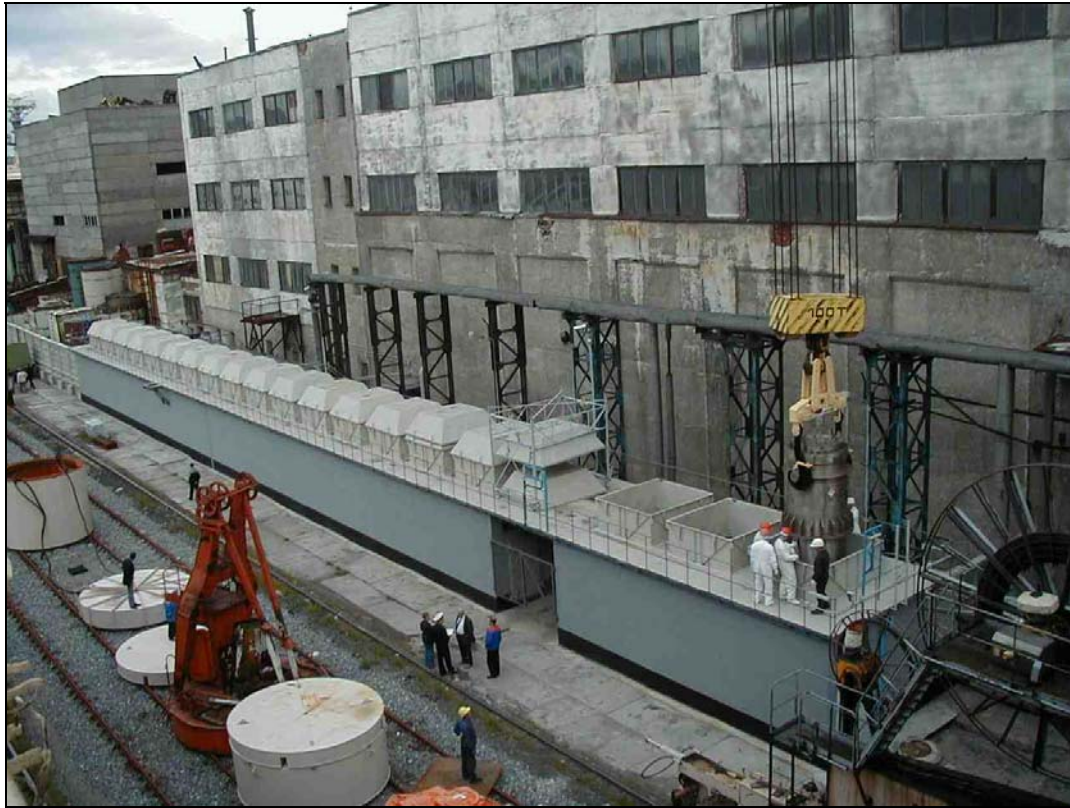
Fig. 3 Hot-testing of the AMEC 1.1-1 Transshipment/Interim Storage Facility at the FGUP “Atomflot” Facility, Murmansk, Russia, August 8, 2003.
